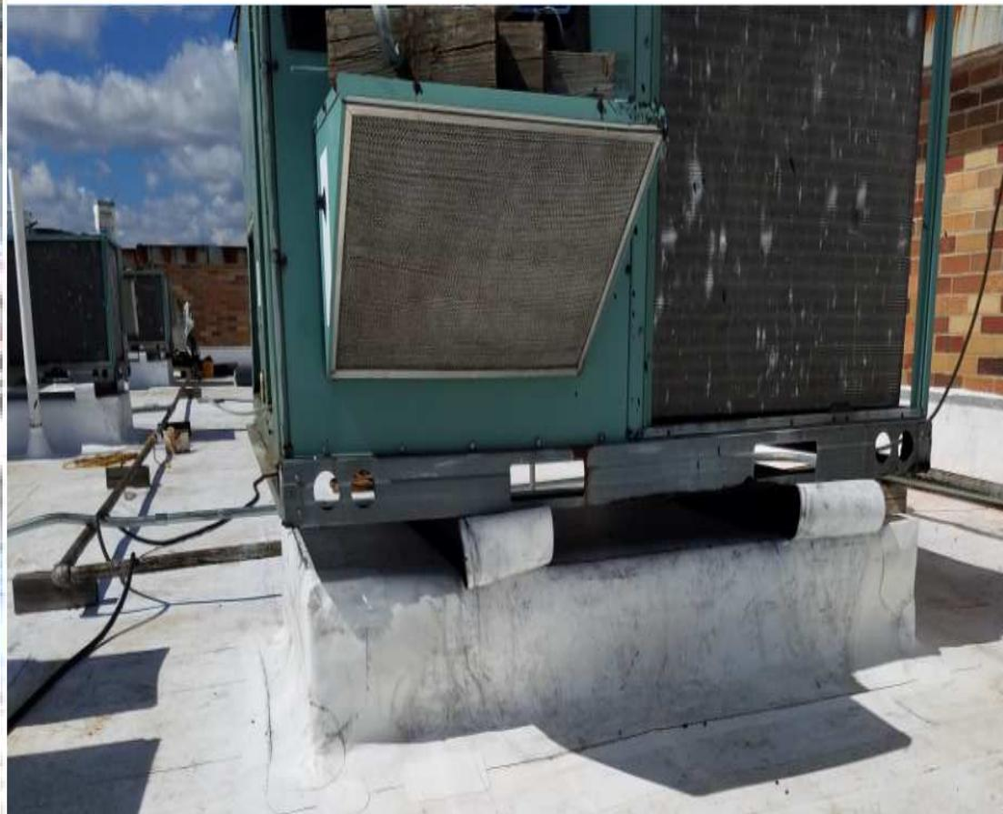
Wet insulation due to condensation from HVAC units
