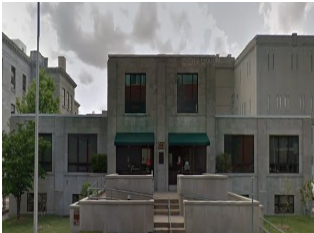
933 N Robberson Facility
